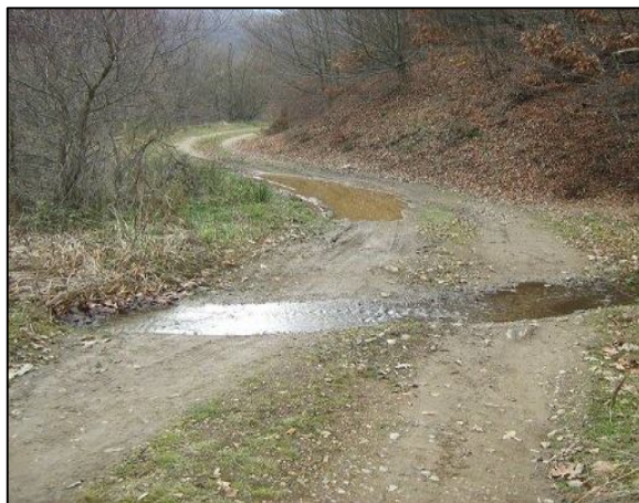
The road before reconstruction
