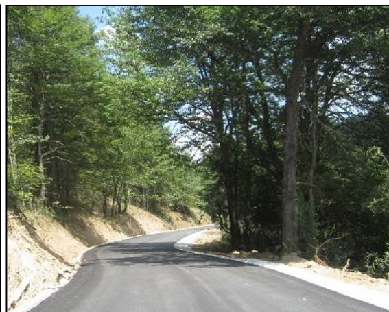
The road after reconstruction
